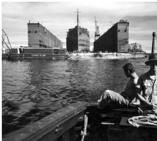
Naval crews were trained in Tiburon on floating auxiliary dry docks that allowed U.S. warships, cruisers and submarines to be repaired out at sea. (Naval History & Heritage Command Collection)
