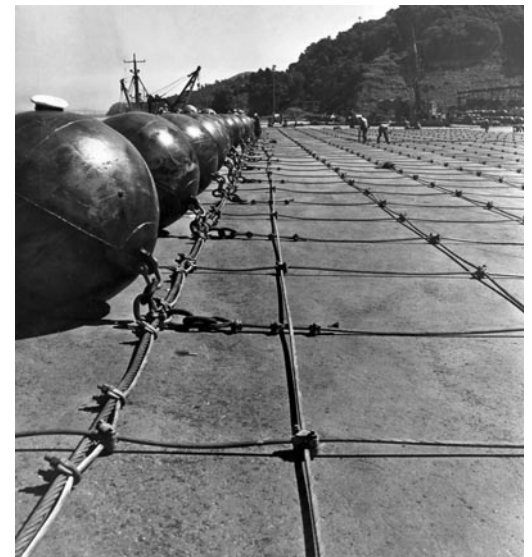
Huge steel antisubmarine nets were constructed on a concrete slab and then pulled off into the Bay and dragged into place by net tenders, with a section that opened to allow friendly ships to enter and depart.
